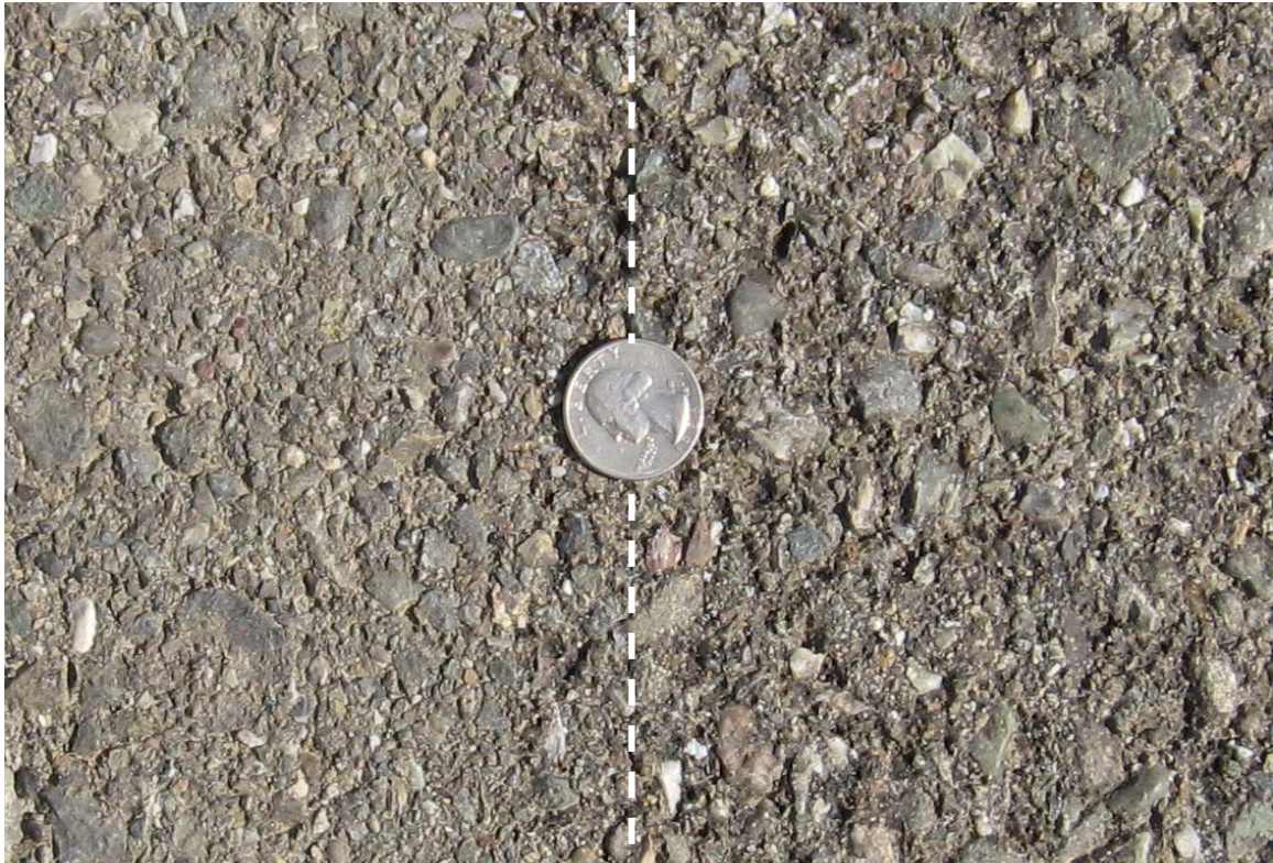
1 2 Figure 3. Surface detail of dense graded asphalt (DGAC) pavement. Left side is 3 original smooth texture. Right side is after retexturing - notice that more fines have 4 been removed, leaving behind larger aggregate.
