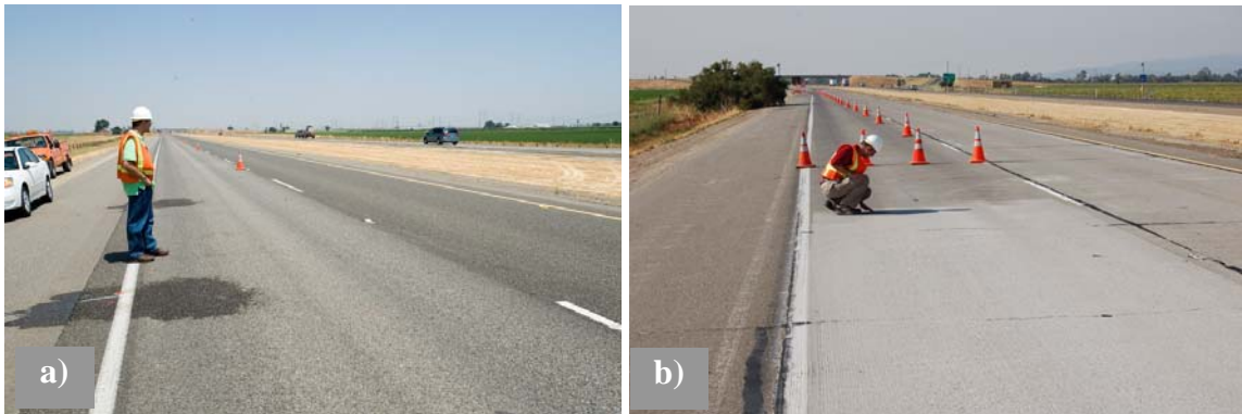
Figure 2. Retextured or ‘skidabraded’ flexible (a) and rigid (b) pavements. After treatment the retextured surface has an elevated friction coefficient and appeared lighter in color than original surface.
