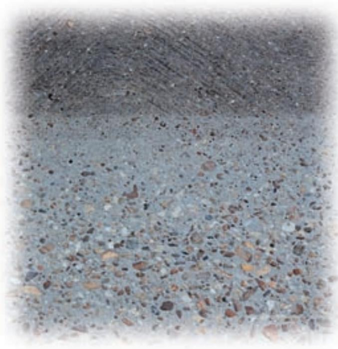
**C**oncrete surface preparation for bonded overlays is easy work for the SKIDABRADER. It removes a controlled amount of bedding mortar and trapped contaminants, and significantly changes the color without leaving machine-produced discolorations or overlap marks. The pores are left clean and open with a microscopic tooth pattern that is essential for maximum bond potential. A production rate of 1,500 to 3,000 square yards per hour per machine is normal for this type of work.
