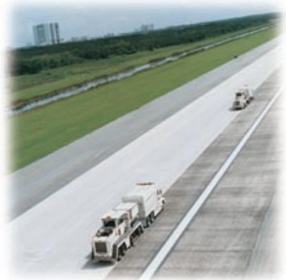
**W**et weather skid resistance can now be applied to most highways, bridges, and airport runways by the SKIDABRADER. The longevity exceeds new pavement.
