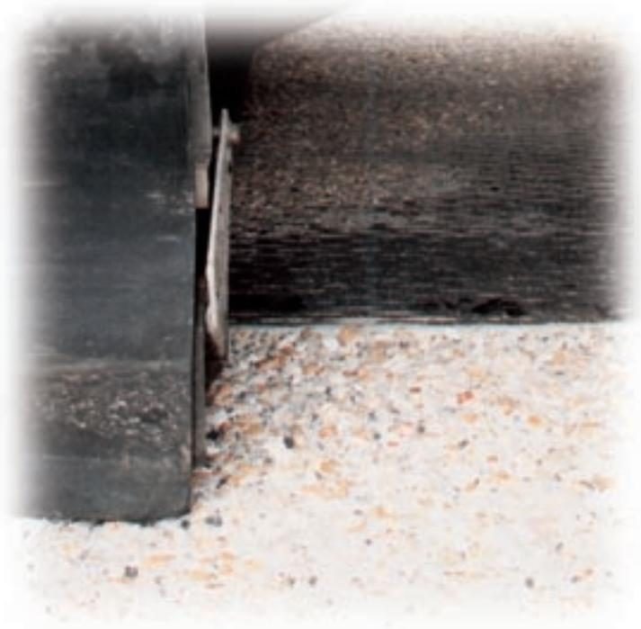
**S**urface depth removal up to 1/2 inch in a single pass can be accomplished safely and cost effective with the SKIDABRADER. There is no cleanup required, and structural integrity is retained. If steel is encountered, it is cleaned and left unharmed. Pre-existing cracks and weak surface mortar have a faster removal rate, and are easily detected. This method provides a highly exposed aggregate, displaying a clean ragged surface for the ultimate bond and overlay interlocking potential.
