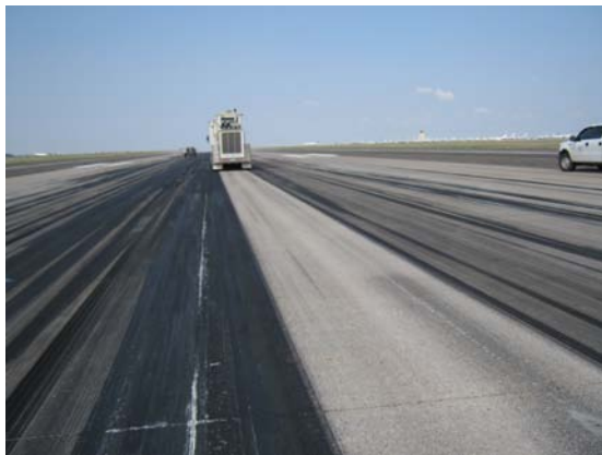
First Skidabrader treatment pass on test section.
